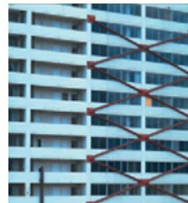
Steel braces will reduce earthquake damage to this concrete building.
